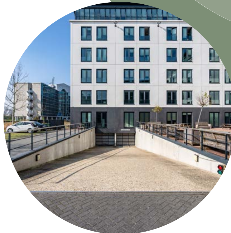
Indoor parking garage
